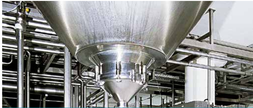
Tank and plant construction
